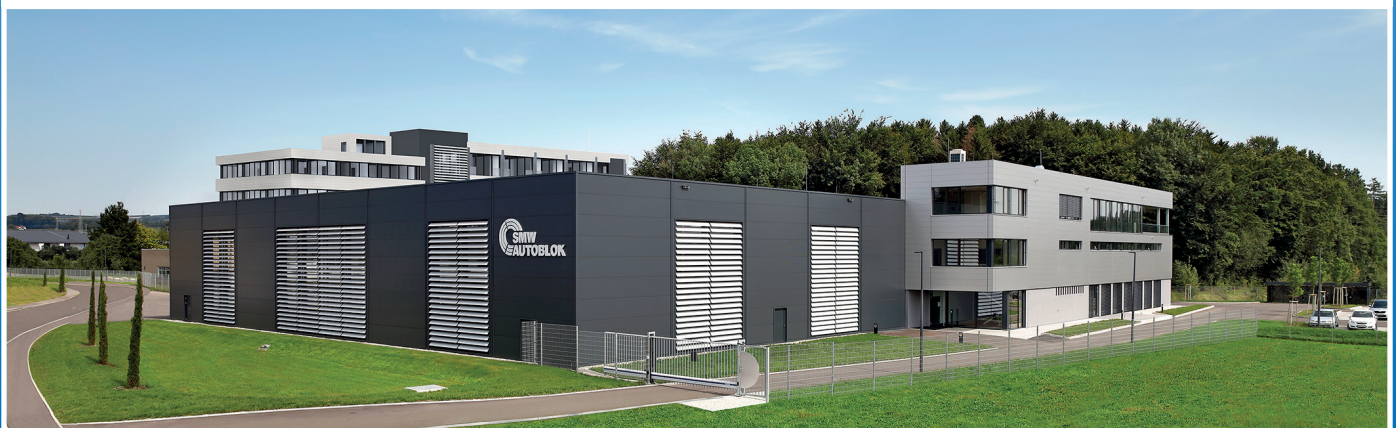
SMW-AUTOBLOK technology and logistics center Meckenbeuren
