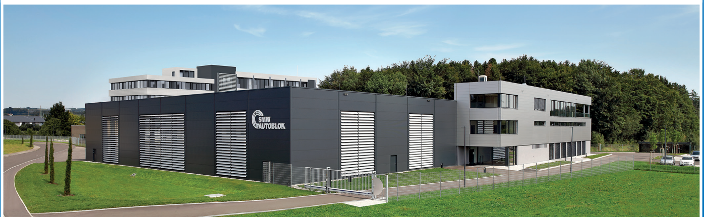
SMW-AUTOBLOK technology and logistics center Meckenbeuren
