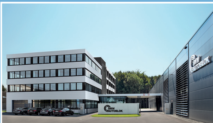
SMW-AUTOBLOK manufacturing plant Meckenbeuren Development | Manufacturing | Sales | Service | Support
