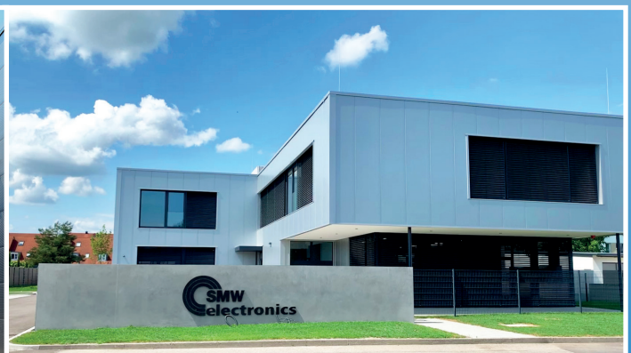
SMW-electronics Meckenbeuren plant Meckenbeuren Development | Manufacturing | Sales | Service | Support
